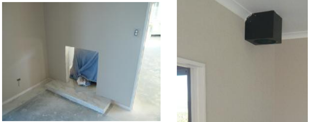
Finished decorated walls and floor protector Flue Drop Box in place
