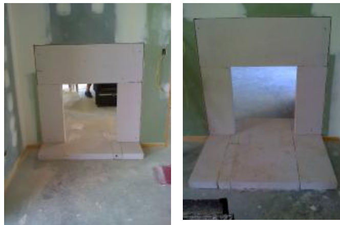
Hebel side and top margin Hebel Floor Protector to flush and freestanding sides
